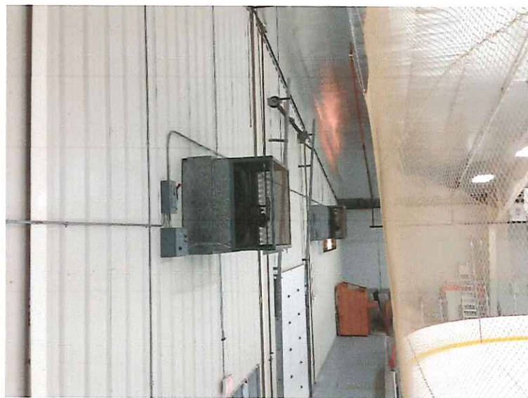
Figure 3-3: Ventilation Fans
