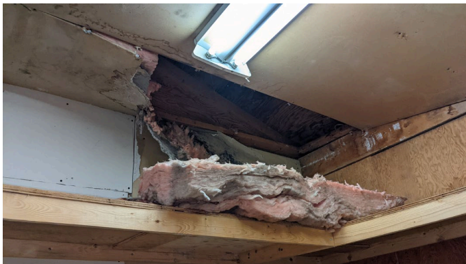
Photo 12: Water Damage & Insulation
