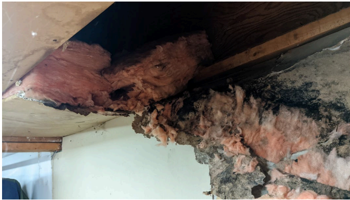
Photo 14: Water & Ceiling Damage
