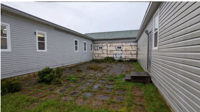
Photo 3: West Elevation (Courtyard) – Wall Damage
