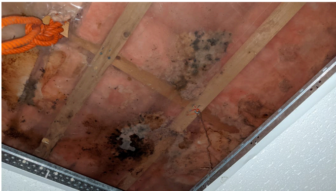
Photo 12: Water Damage & Insulation
