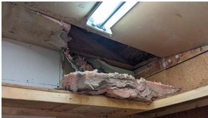
Photo 12: Water Damage & Insulation
