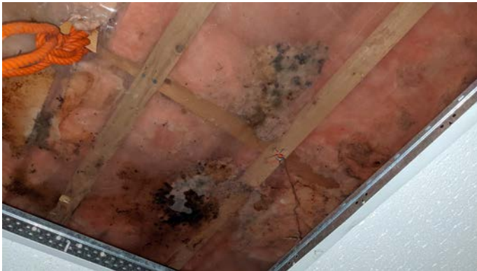
Photo 12: Water Damage & Insulation
